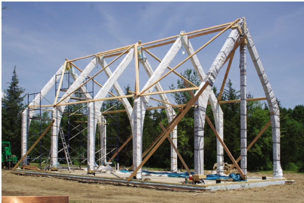
FIVE GLU-LAM TRUSSES FRAME THE HUDSON PASSIVE HOUSE, DESIGNED TO USE 90 PERCENT LESS HEATING ENERGY THAN A TYPICAL THREE-BEDROOM HOUSE JOHN ISAACS
