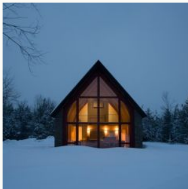
The large glass wall at the south end of the house lets the... More >
