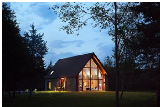
By virtue of its forward-thinking design and construction, New York State's first passive house — located in Columbia County — practically heats itself
