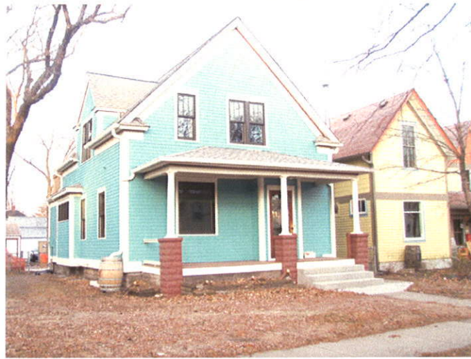
Deep energy-efficient retrofit using retrofit insulated panels by Panelworks Plus
