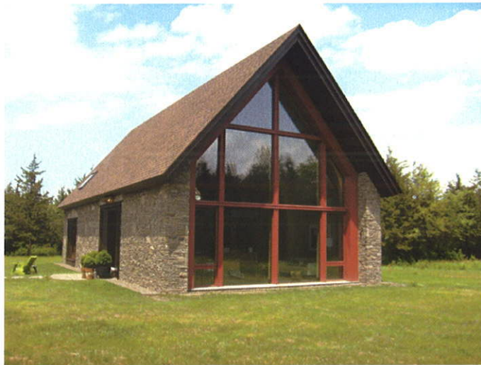
Hudson Passive Project by Timberline Panel Company
