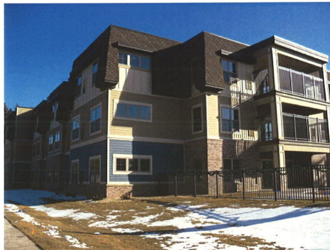
Coventry Senior Living complex by Energy Panel Structures
